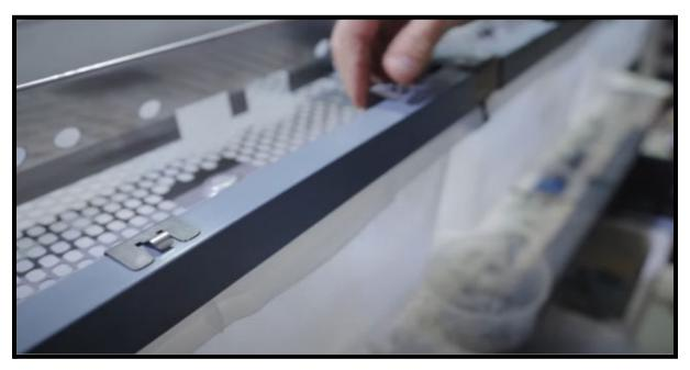
(Waterline clips attach over the back of the vent clips, with the clip opening facing forward.)
